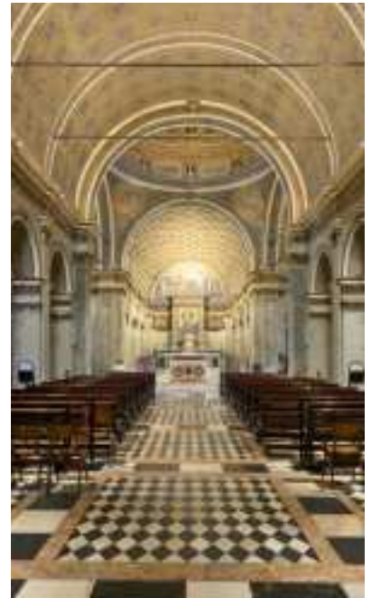
Up: Basilica di Santa Maria presso San Satiro New lighting project by Giorgio Ripa - Area Studio S.r.l. Milan (Italy)
