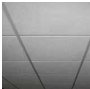
SUSPENDED T-BAR & CEILING TILES (MIN. 8 MM)
