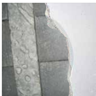
CONCRETE BEAM & BLOCK + PLASTER
