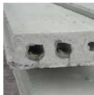
PREFABRICATED CONCRETE PLATE + PLASTER
