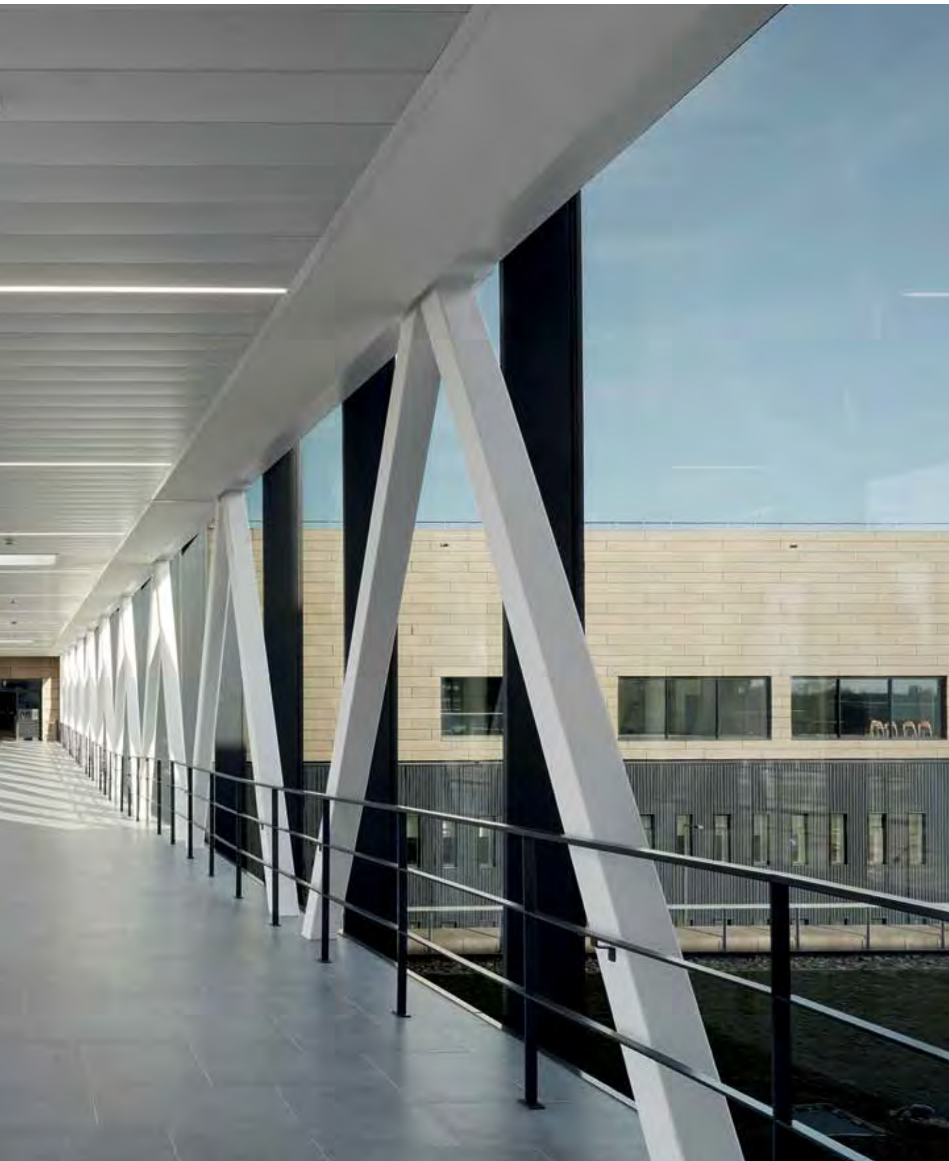
PROJECT AZ DELTA GENERAL HOSPITAL ROESELARE CAMPUS / ARCHITECT VK ARCHITECTS & ENGINEERS / INSTALLATION EEG GROUP
