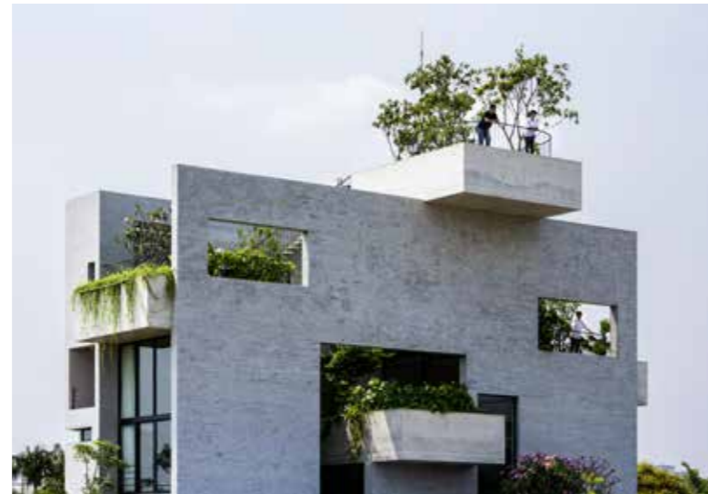
Im Binh House in Ho-Chi-Minh-Stadt bilden Pflanzen eine Art natürlicher Klimaanlage. In Binh House in Ho Chi Minh City, plants act as a kind of natural air-conditioning. (Vo Trong Nghia Architects)
