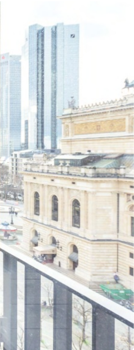
Satellite Office Opernplatz Frankfurt, Germany Cubic W4 Photography: Moritz Bernouly, www.satelliteoffice.de
