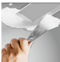
skimmed into plasterboard ceiling (trimless)
