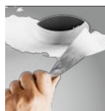
skimmed into plasterboard ceiling (trimless)
