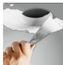
skimmed into plasterboard ceiling (trimless)
