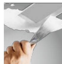
skimmed into plasterboard ceiling (trimless)
