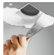
skimmed into plasterboard ceiling (trimless)
