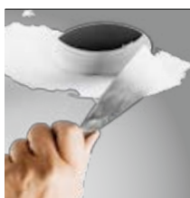
skimmed into plasterboard ceiling (trimless)
