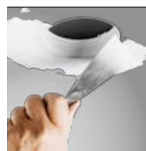
skimmed into plasterboard ceiling (trimless)
