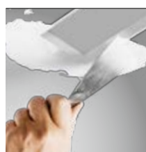
skimmed into plasterboard ceiling (trimless)
