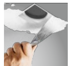
skimmed into plasterboard ceiling (trimless)
