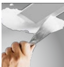
skimmed into plasterboard ceiling (trimless)
