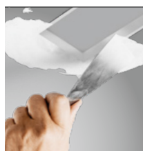
skimmed into plasterboard ceiling (trimless)
